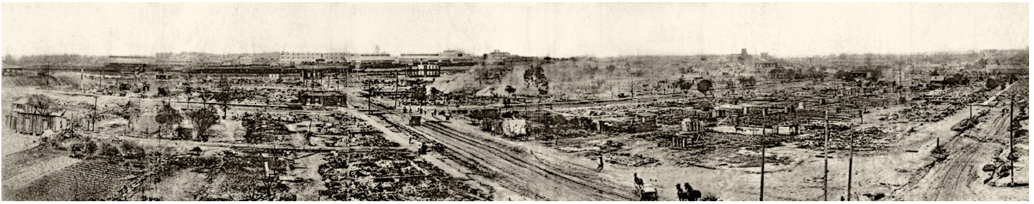
THIS photograph was taken from the roof of Booker T. Washington High School and reveals much of the damage that occurred within a day or so of the Tulsa massacre of 1921. The road running east to west (laterally across) through the center of the photo is Greenwood Avenue .
