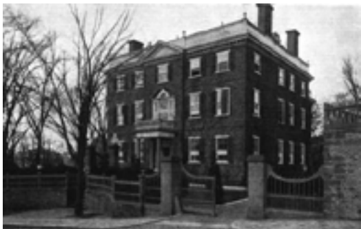
home of John Brown, slave trader, on Benefit Street in Providence, Rhode Island.
