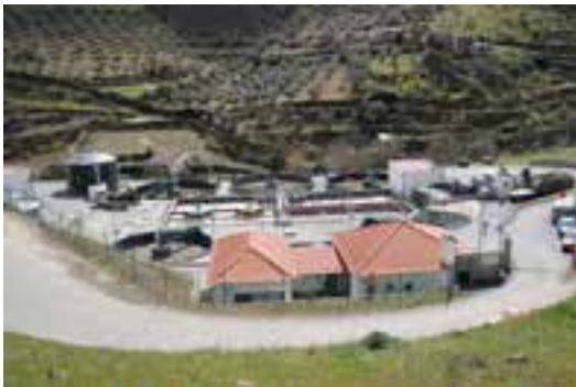
photo of a sewage treatment facility in Portugal owned and operated by Veolia. Veolia is the water division of the French company, Veolia Environment, and the world's largest supplier of water services.
