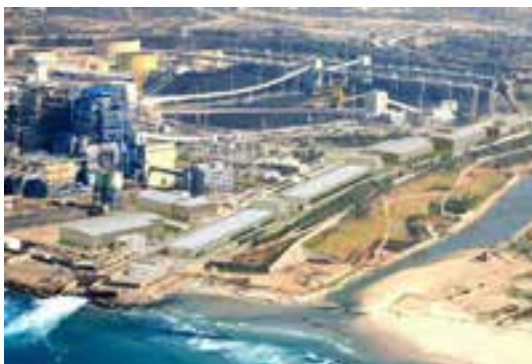
Israeli Desalination plant
